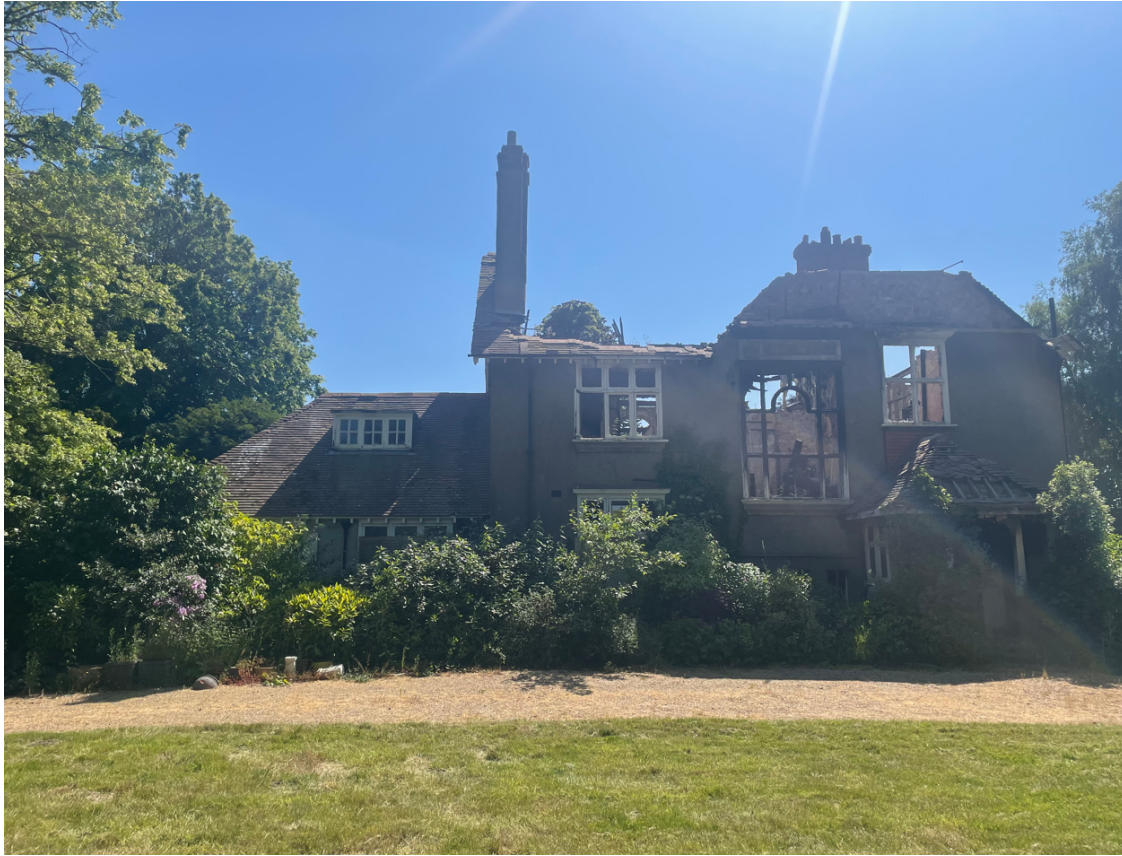
Figure 3: Existing Dwelling – Front Elevation
